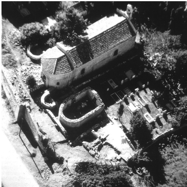
Fig. 25. Osor. The Cathedral Church of St. Mary (Aerial View)
